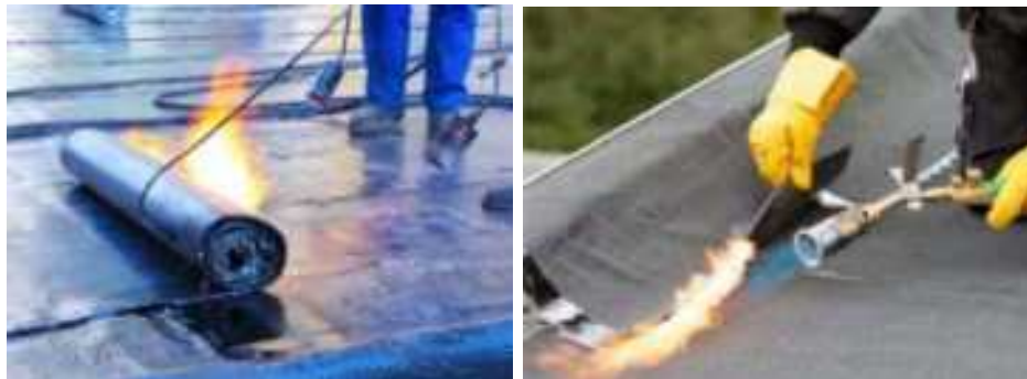
Fig. 4. The installation process of adhesive waterproofing materials
